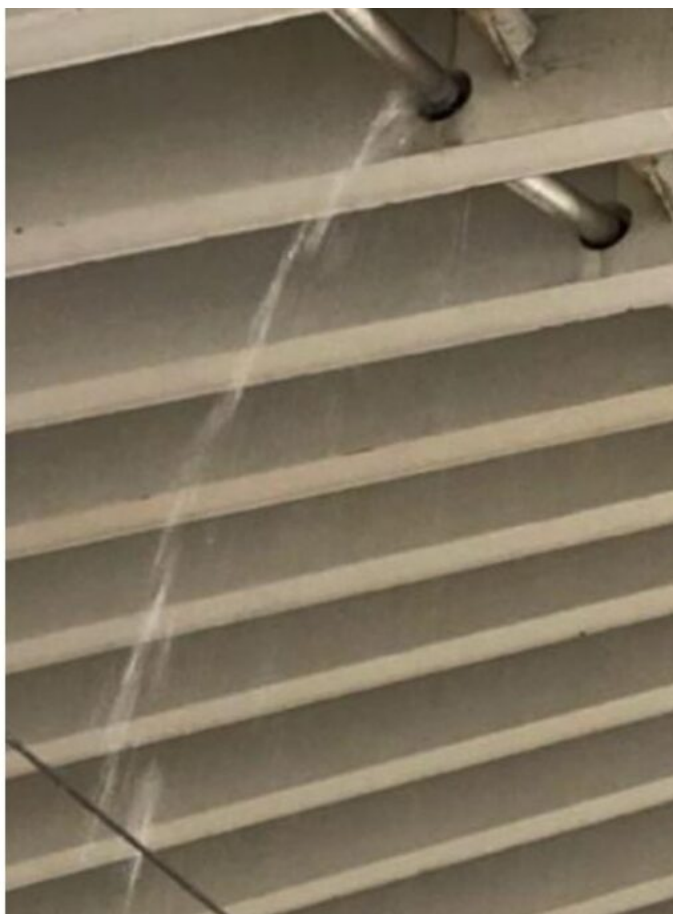
a) An image of the flooded platform. b) Rainwater leaking from one of the drainage pipes running through the vault (photo credits Augusto Giuffredi).
