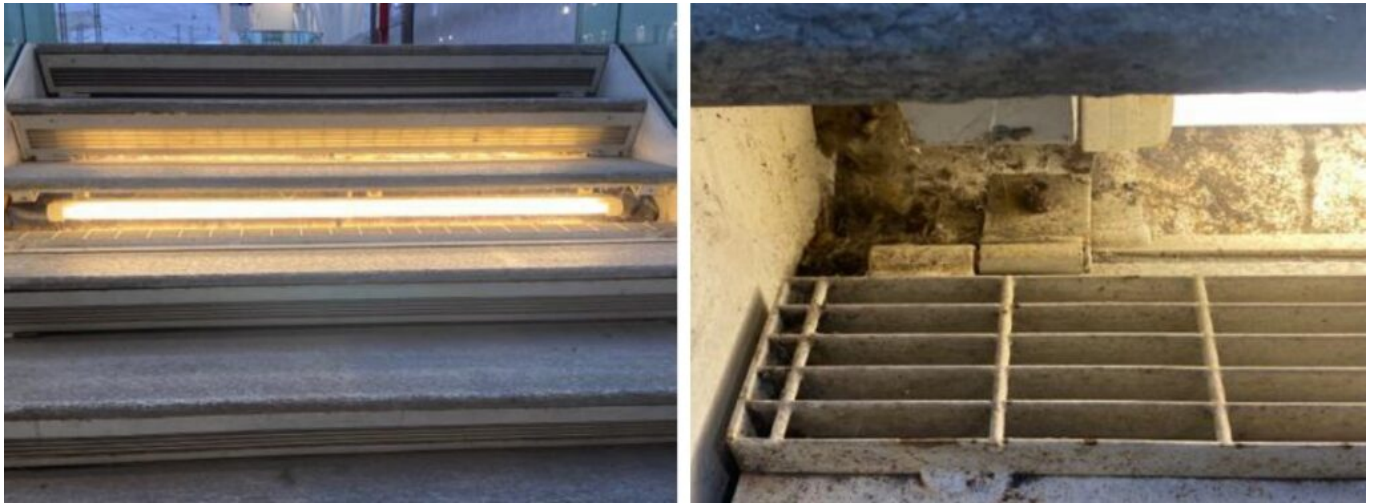
a) Steps of a track access staircase. b) Detail of the riser of a step with an open grid for maintenance (photo credits Augusto Giuffredi).
