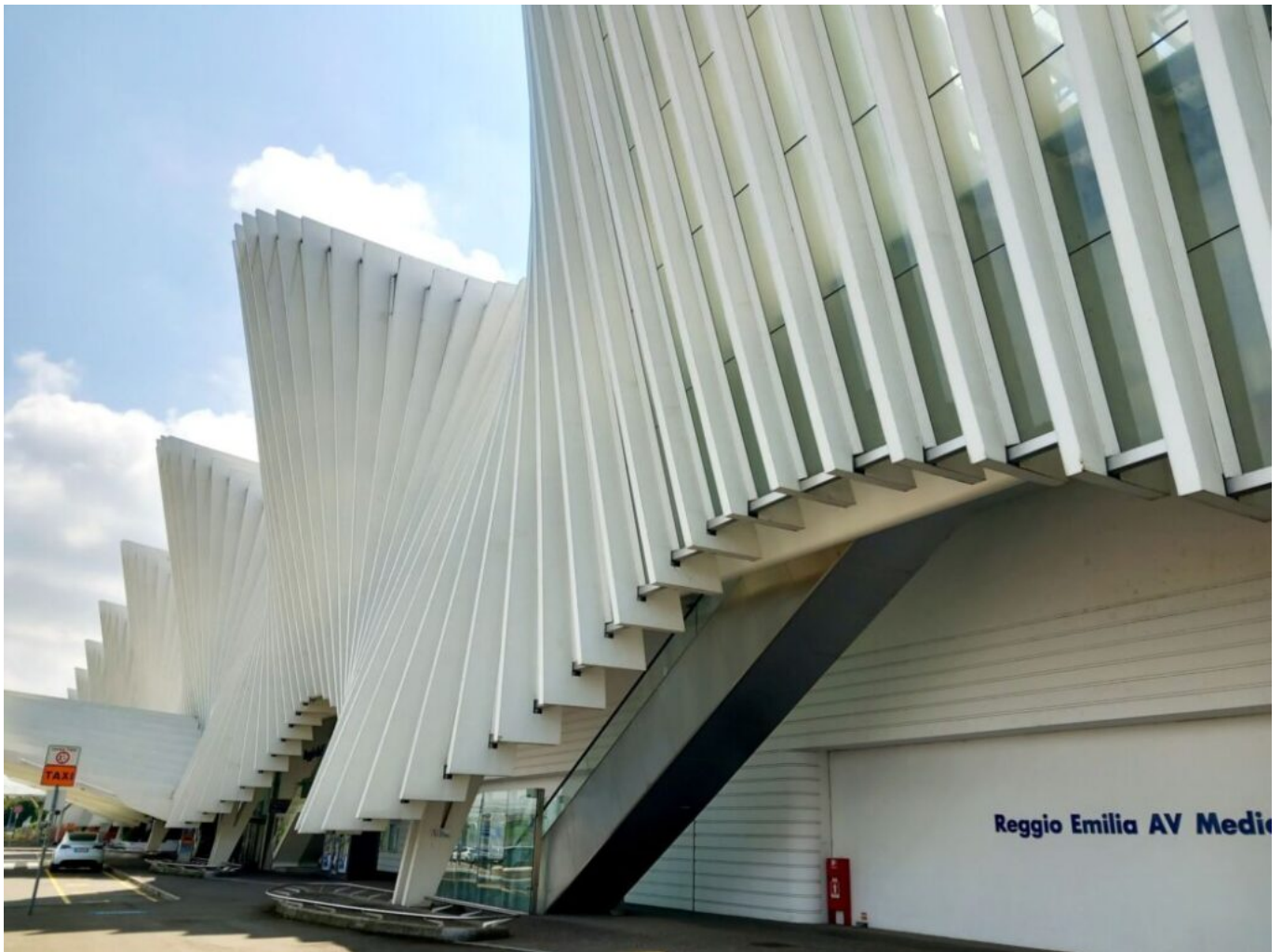
Exterior of the Mediopadana station on the car park side, with in the foreground one of the elevations with anti-slip bollards installed after the inauguration ( www.24emilia.com ).
